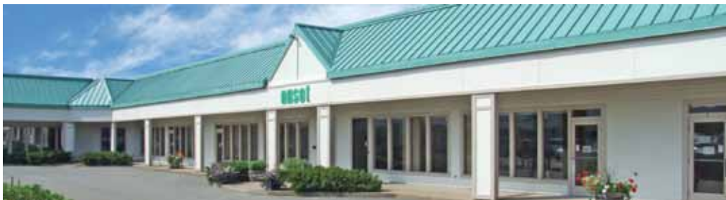
Onset headquarters, Cape Cod, MA
