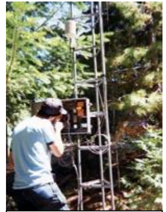
Weather Station being installed on 130 ft. Triangular Instrument Tower
